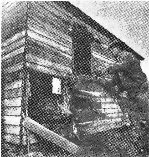
END OF AN ERA? Another farm labor cabin burns.
